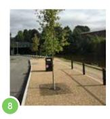
Before the pavement is finished, construct the tree pit curbing. Any type of shape or finish to engineers' specification can be used. The tree pit can also be left open for optimal aeration and irrigation.
