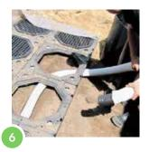
Do not completely fill the system – leave an aeration layer directly beneath the top frame of 50-100mm.
