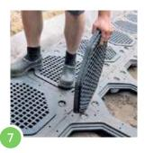
Finally, seal the system with the decks and cover. Drop in the inspection/aeration decks and cover with the final separation geo-textile to prevent any of the buildup dropping into the tree pit. These can also be used as inspection hatches. The system is ideal for use underneath a permeable top surface.
