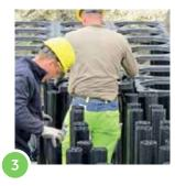
After all the base frames are in position, the support posts and top frames are installed, straddling any service lines as required. The posts are available in six height options and can also be manually adjusted as work is in progress, to overcome any unexpected underground obstacles.
