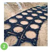
The base frames are installed according to the layout plan, leaving 30cm working room around the edge of the units. The units can be installed with a spacing of up to 75mm; this means that curved installations and non-standard dimensions are possible. Dimensions of a single unit are 605 x 605mm.
