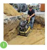
The first stage is to ensure the base of your tree pit is level and consolidated to your engineer's specification. Getting this right is crucial to the success of the tree pit.
