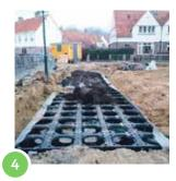
After all the units have been installed the system is enclosed by the reinforced separation. This can be backed by an additional permeable root barrier if required.
