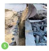
The system is now ready to be filled. Backfill the surrounding trench then the inside of the tree pit, alternately in 200-300mm layers. Maximum compaction for the backfill is important, manually consolidate the soil inside the system by foot, ensuring maximum soil volume for the tree.
