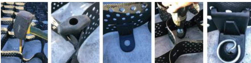
Steel Pins Plastic Pin Caps CellGrip Fixing Install with Drill Finished
